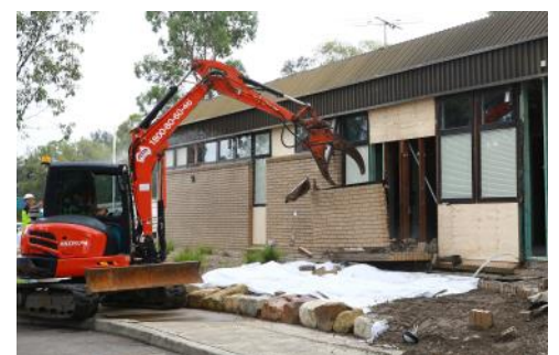
▲ Admin building demolition underway
